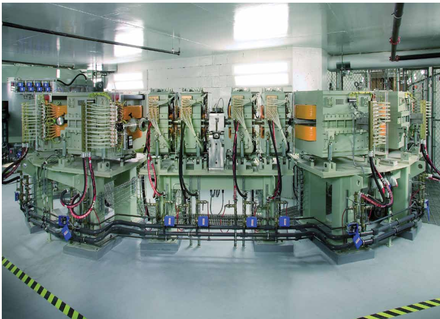
Fig. 5: View on beamline and cyclotron (reference: iba)
