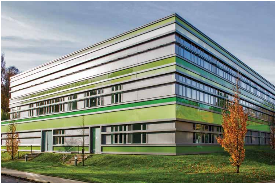
Fig. 4: Building of the WPE facility (reference: WPE)
